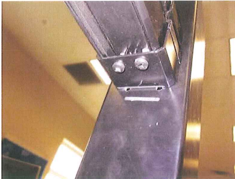
Photo No. 6 Top Rail Bracket-to-Rail Connection
