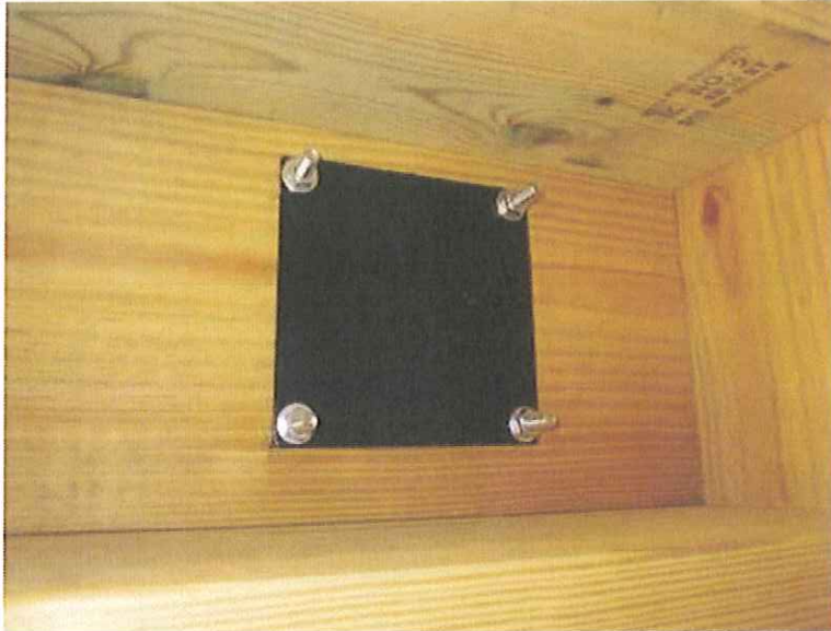
Photo No. 5 Post Mount Attached to Mock Wood Deck
