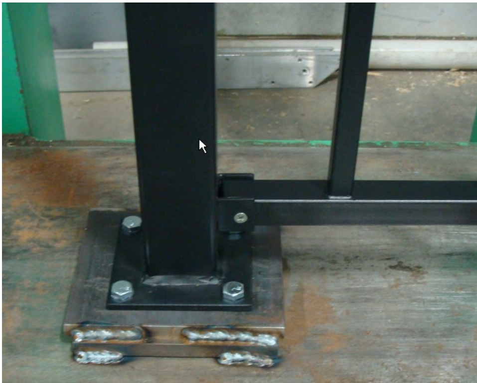
PHOTO 2: Post Mounted on to Test Frame
