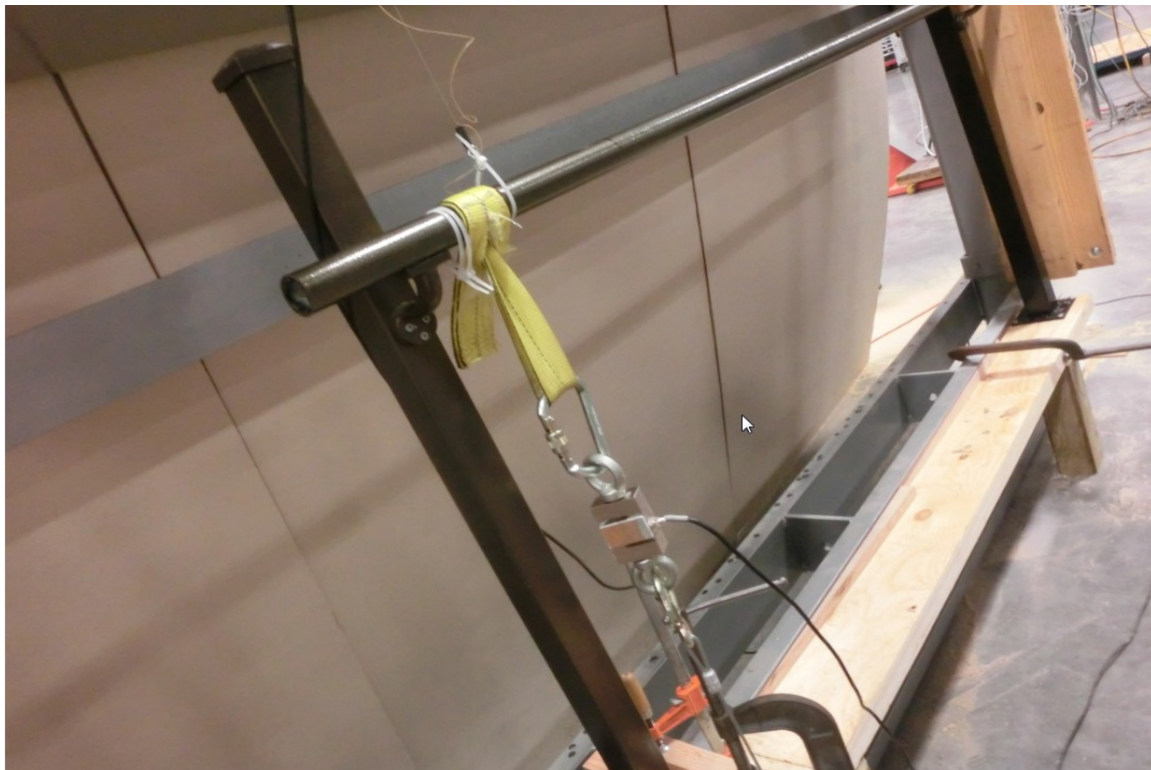
Photo 10: Typical Setup for Vertical Concentrated Load Near Support
