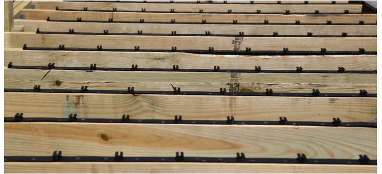
Strips may be installed on joists all at once prior to installing decking or one row at a time for elevated decks.
