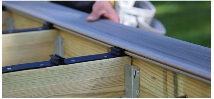
Slide starter board tightly into first set of clips and secure with composite deck screws along the outer edge of board.
